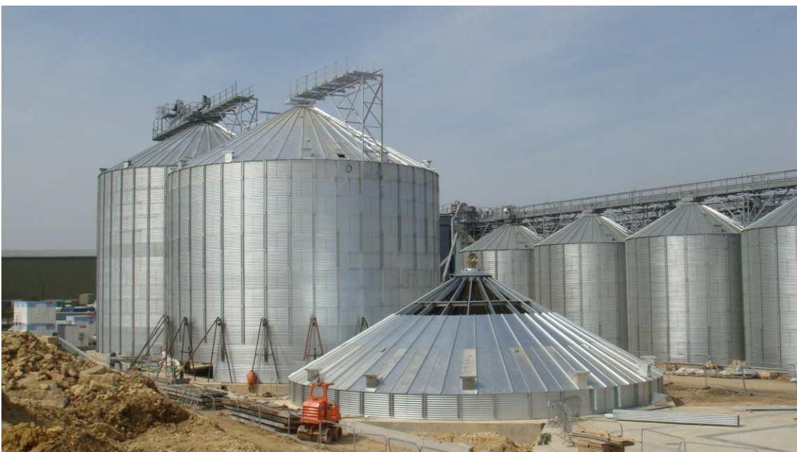
G2 Silo works barrel progressing along with G3 roof.
