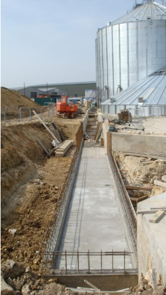
Discharge channel progressing
